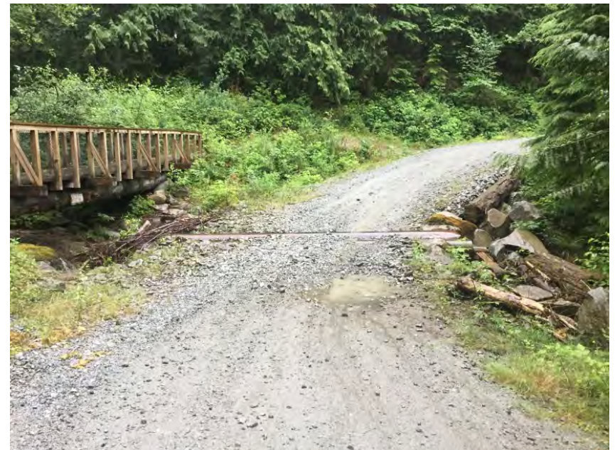
Approach from Right Bank when facing downstream
